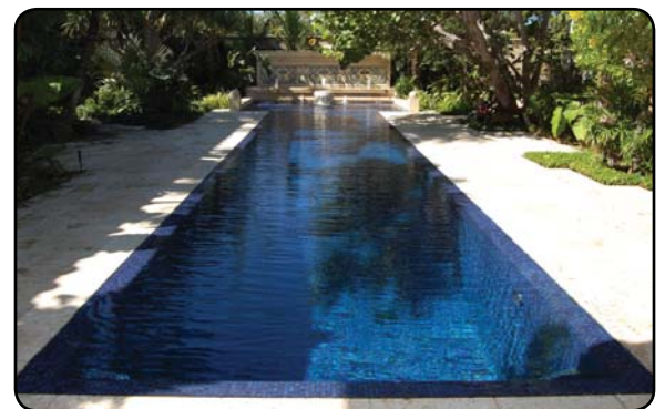
Gold - Hackl Pool Construction Co., Inc.
